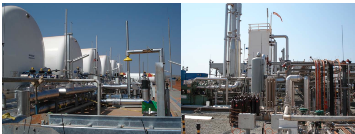
Figure 21. EDL virtual pipeline facility: LNG storage tanks (left) and cold box unit (right).
